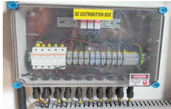
Fig. 5 Installed DCDB
